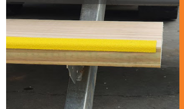
STEEL STRINGERS AND TIMBER TREADS
